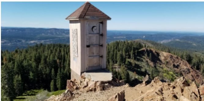
High Altitude Bathroom Structure
